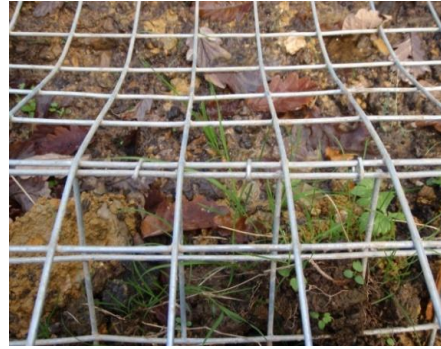
Figure 21. Hog rings connecting fencing.
