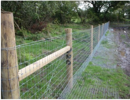
Figure 20. Standard beaver fencing to discourage digging and gnawing.
