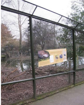
Figures 14 & 15. Different perimeter fencing used to retain beavers at RZSS Edinburgh Zoo (left) and Highland Wildlife Park (right).
